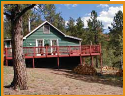
Figure 10: Decks, exterior walls and windows are important areas to examine when addressing structure ignitability. Photo: CSFS
