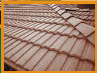
Figure 9: (above right) Class A roofing materials including tile, clay, concrete, slate and asphalt shingles are fire-resistant options. Photo: CSFS
